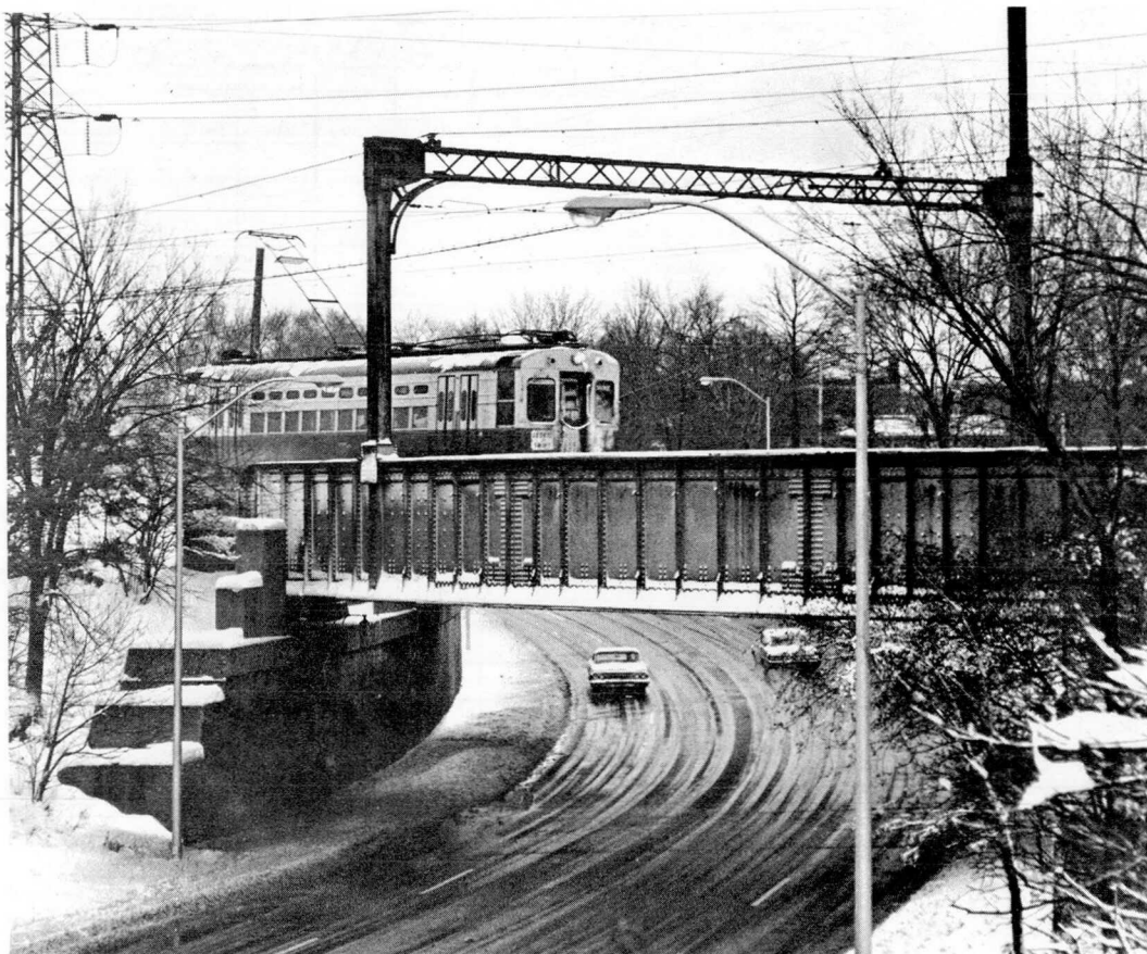
Mornings like this one helped to popularize Skokie Swift's freedom from street traffic. The train pictured here is on the Skokie Boulevard overpass, the only grade-separated crossing on the Swift route in the Village of Skokie.
