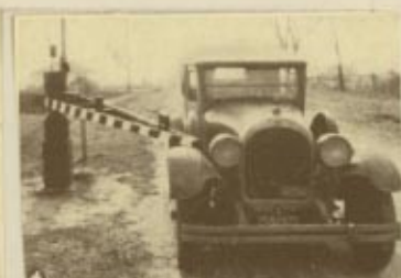
(4) Gate being swung aside by automobile failing to stop
