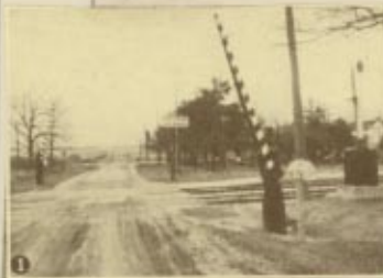
(1) The gate when not in operation
