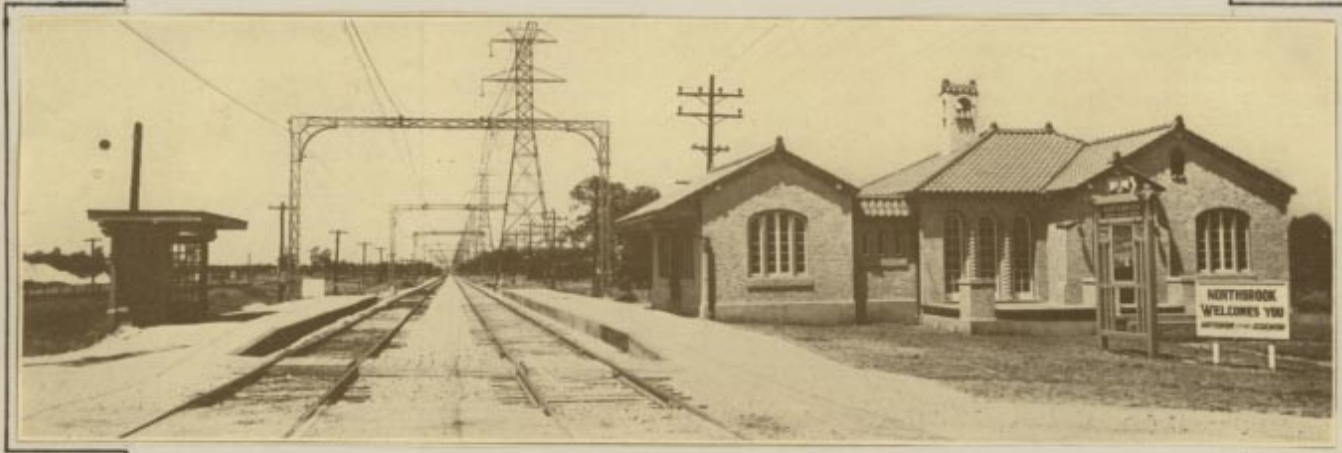
Steel Tower Catenary and Northbrook Station on the North Shore Line in 1924
