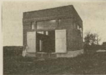
Automatic Substation, Winthrop Harbor, North Shore Line
