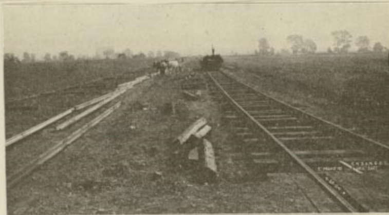
Laying permanent track on Niles Center Extension
