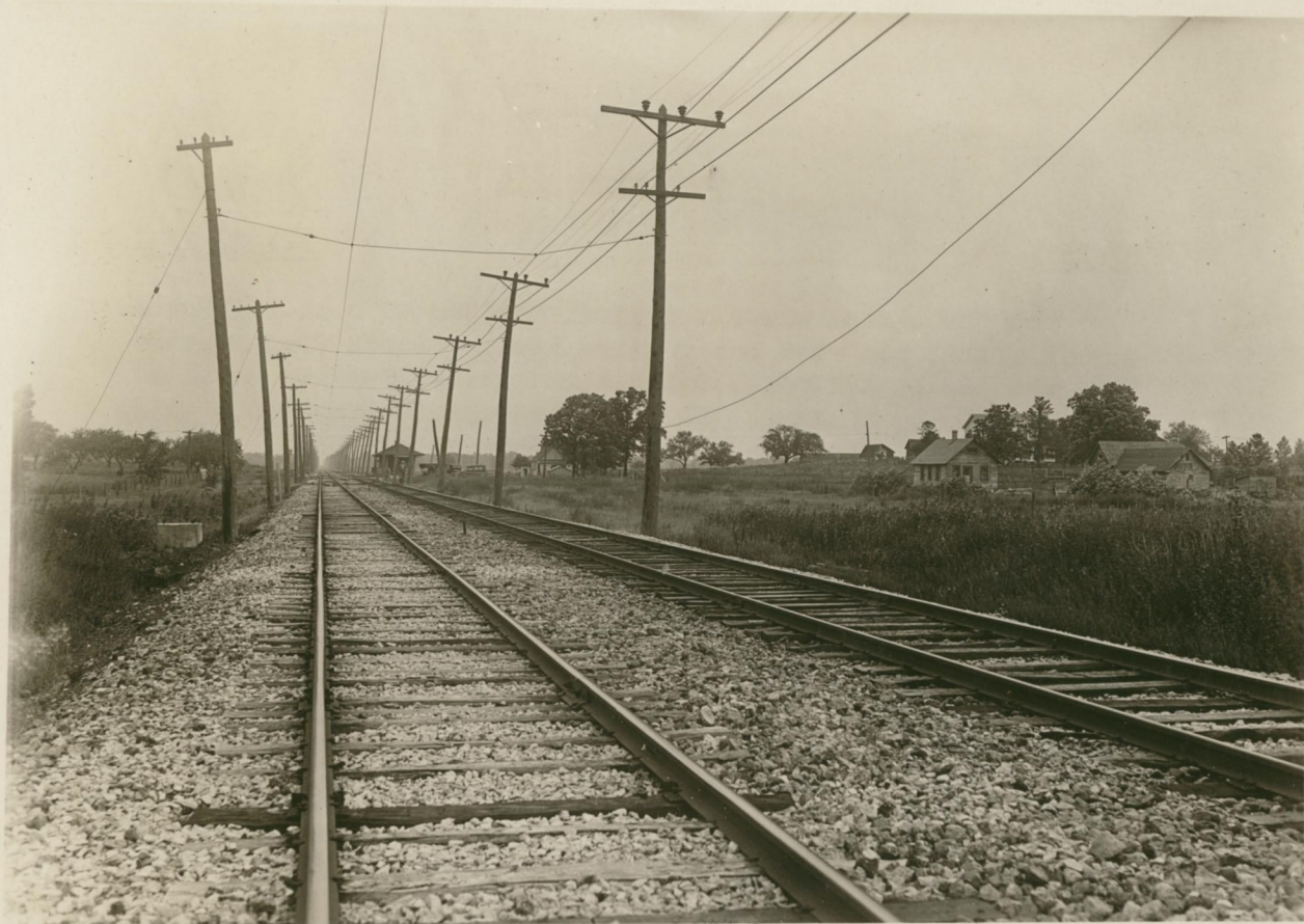
Section of rock-ballasted double track, looking north from a point near the Beach, Illinois, substation, about 38 miles north of the Union Loop, Chicago, in July, 1924. Much of the Company track is of this character, the ballast extending to a depth of about 10 inches beneath the tie, and is obtained principally from a quarry about two miles north of Racine, Wisconsin.
