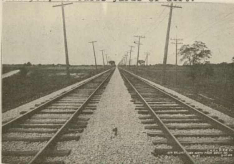
Completed stone-ballasted track on top of solid fill which replaces former open trestle work
