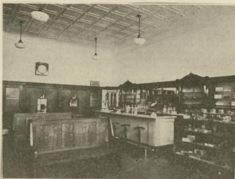
Interior view of New North Shore Line Station Lake Geneva, Wisc.
