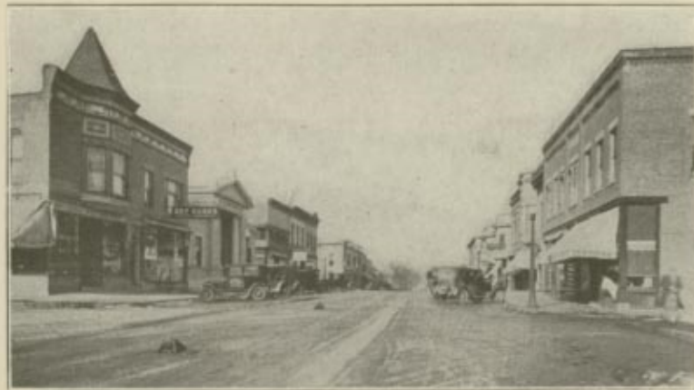
A View of Libertyville's Business Section -1926
