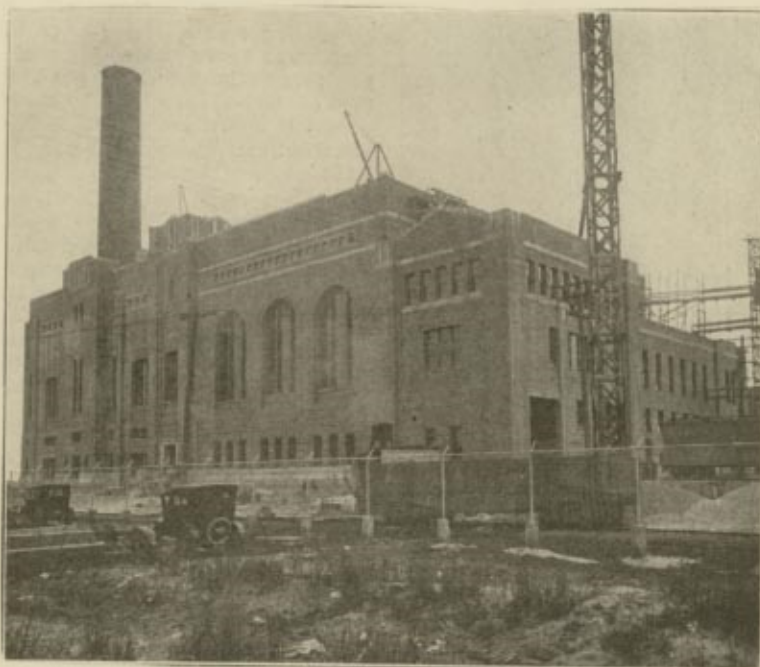
Plant of Public Service Company Waukegan, Illinois
