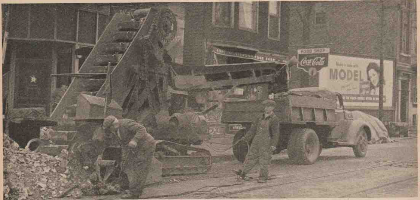
STREET CLEANERS: Removal of excavated material is handled with an electrically operated bucket loader, a great improvement over the old hand-shoveling method. All but the very
