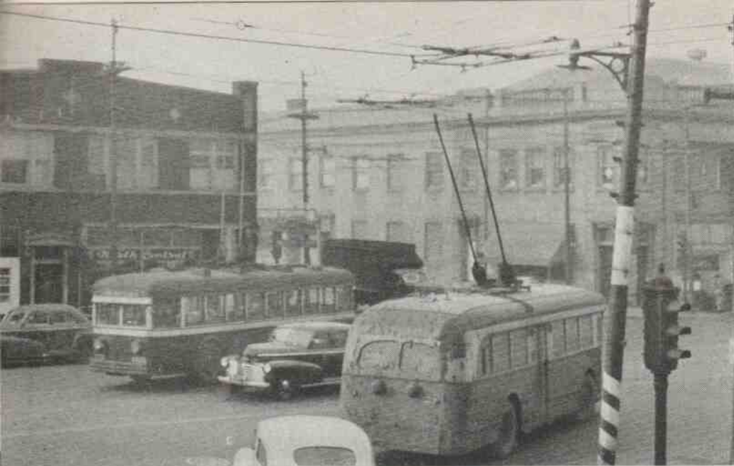
Simplified overhead at Central and North eliminates an accident hazard by widening the spread between bus lanes—permitting the free passage of auto traffic between buses on the "S" curve.
