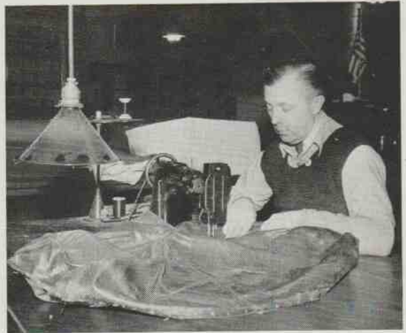
Frank Porcaro (Carpenter Shop) removes a slashed seat cover while Joseph VanDerhaeghen (Curtain Shop) sews a new piece of leather into a damaged seat. (Pictures taken at West Shops).
