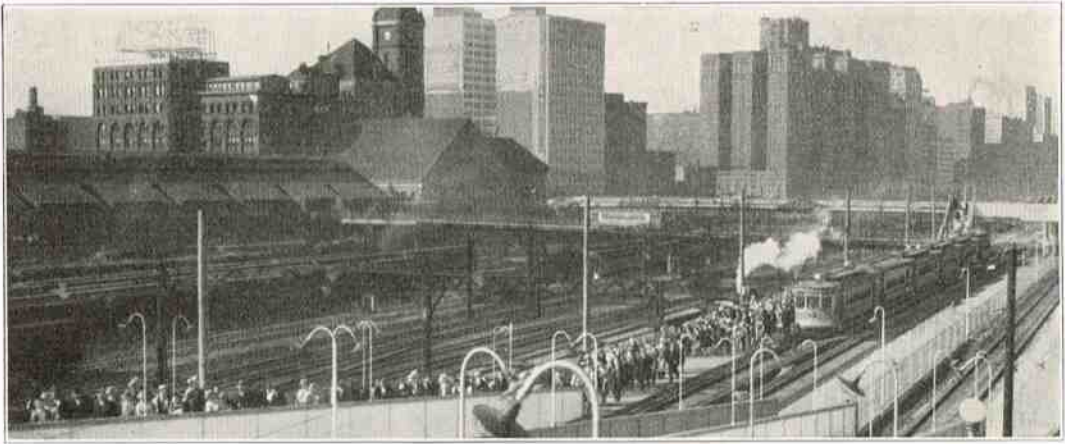
Bringing the Crowds in at the North Gate Terminal
