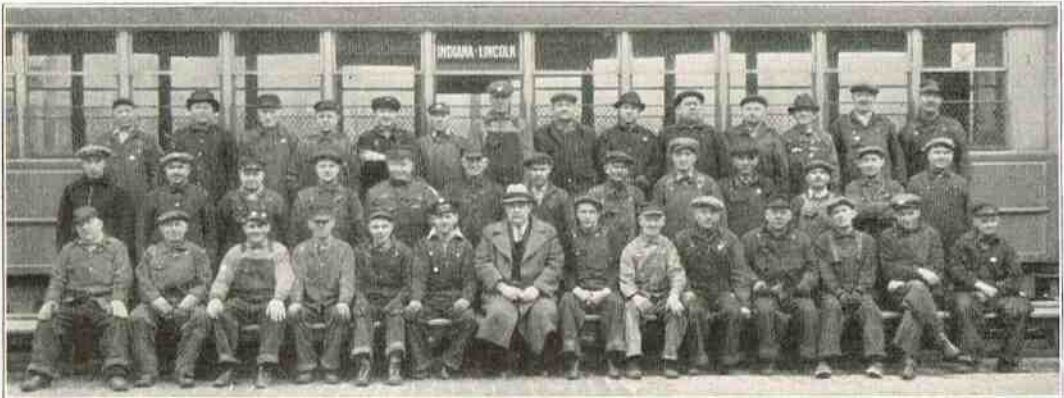
Cottage Grove Pull-in Crew
