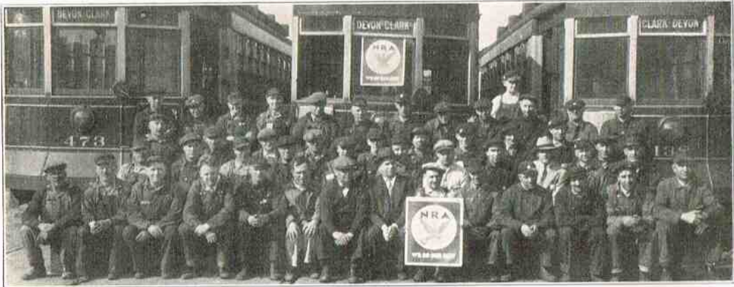
Devon Carhouse Pull-In Crew
