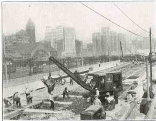
Advance Work East of the Illinois Central Tracks.
