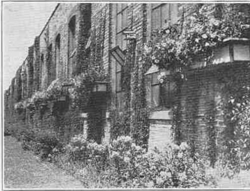
The South Wall at Devon Transformed by Vine and Blossom
