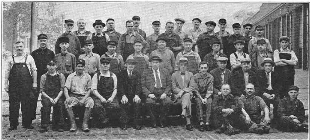
Cottage Grove Winning Repair Crew
