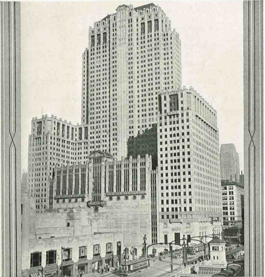
LOOKING NORTHEAST ACROSS MADISON STREET BRIDGE TO THE CIVIC OPERA HOUSE
