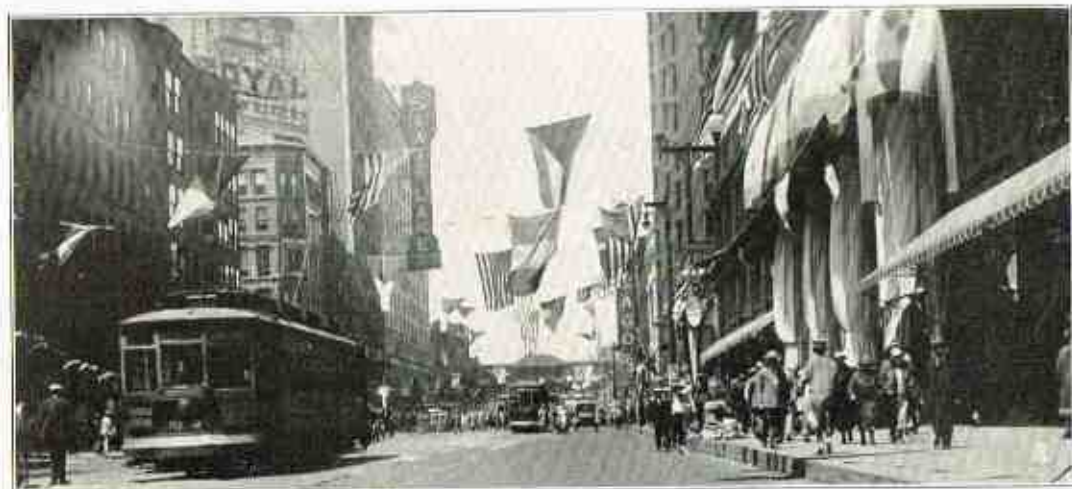
What "No Parking" Means—State Street Looking North from Washington Street
