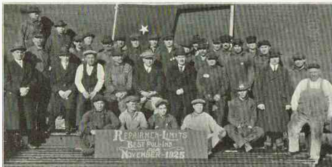
The Limits Car House Repair Crew
